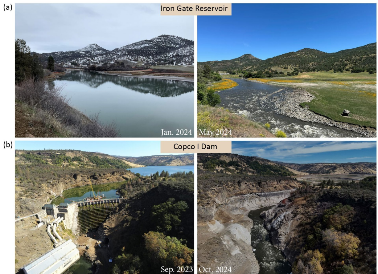
Fig. 2. Images of before and after dam removal on the Klamath River. (A1) Upstream view of the Iron Gate Reservoir below Fall Creek, prior to the start of reservoir drawdown and dam removal, beginning of January 2024 (Photo credit: resource environmental solutions (RES)). (A2) Same location as (A1) , now an upstream view of the Klamath River below Fall Creek, taken within the former Iron Gate Reservoir footprint, May 2024 (Photo credit: RES). (B1) Drone image of the Copco 1 Dam, completed in 1918, along the Klamath River during pre-dam removal activities in September 2023 (Photo credit: RES). (B2) Drone image of the Klamath River at the former Copco 1 Dam site following the completion of dam removal activities in October 2024 (Photo credit: RES).
